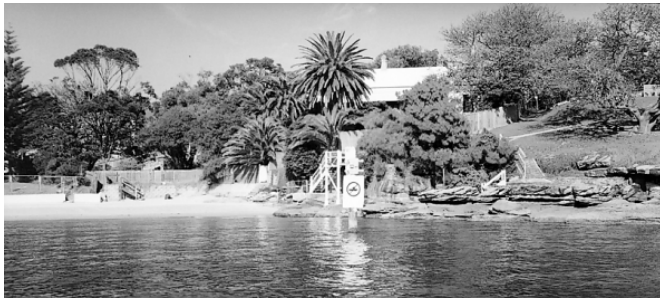
Former Marine Biological Research Station at Green (Laings) Point
