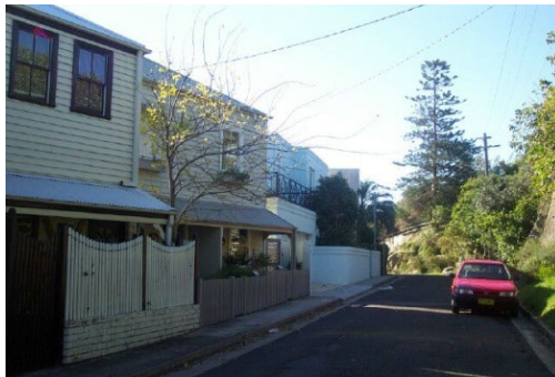
FIGURE 30 Group of two storey Victorian timber cottages on Gap Road
