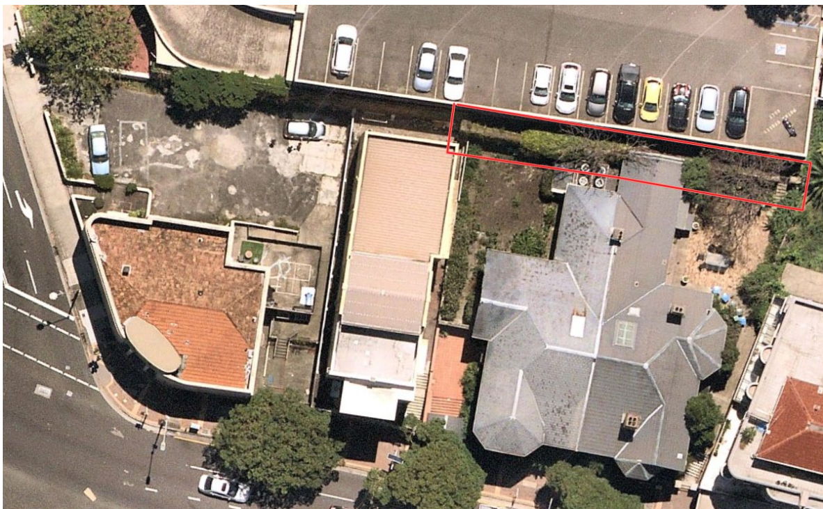
Figure 6 – Location of retaining wall and stairs on the northern boundary of the site
