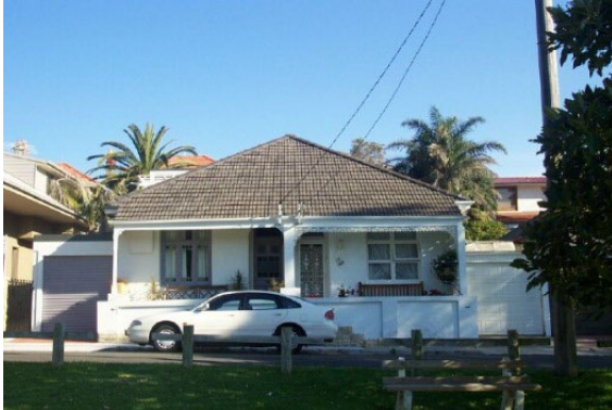
FIGURE 39 One of three pairs of single storey semis
