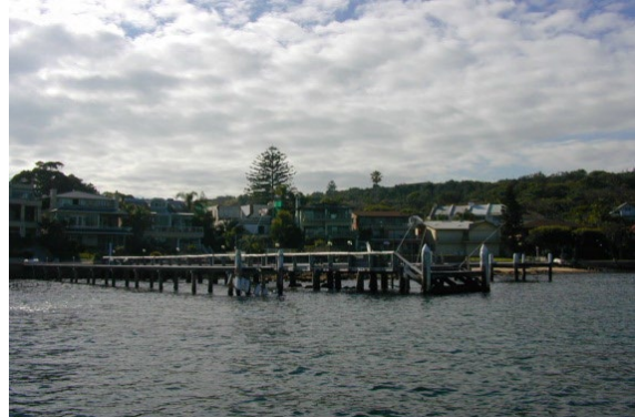
FIGURE 65 Jetties within the Pacific Street Precinct, extending out over rockshelves
