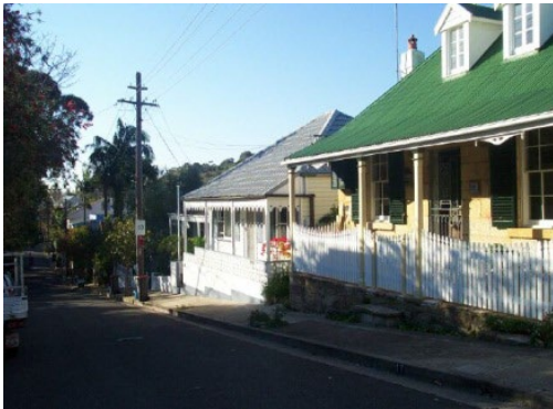
FIGURE 79 Stone and weatherboard cottages on Cove Street
