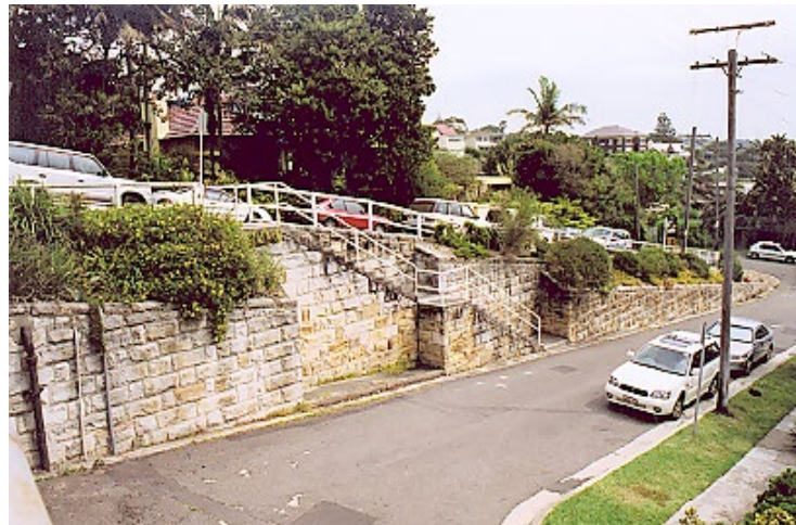
Sandstone retaining wall along Salisbury Street
