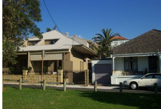
FIGURE 40 One of three pairs of single storey semis
