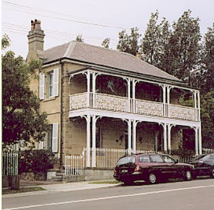
FIGURE 10 Contributory item on Old South Head Road illustrating dominant materials, including sandstone blockwork and slate roofing.
