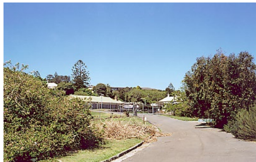
FIGURE 149 HMAS Watson within its setting of native vegetation and cultural plantings
