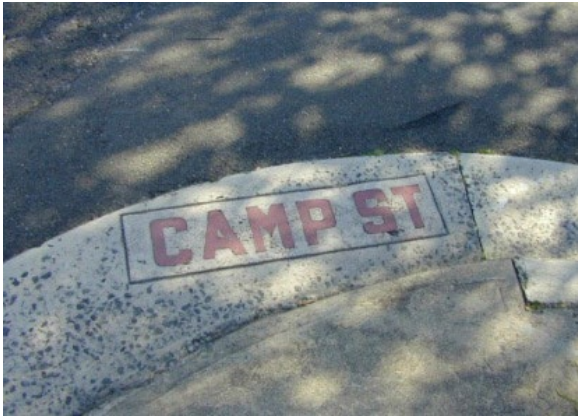
Camp Street name incorporated into gutter
