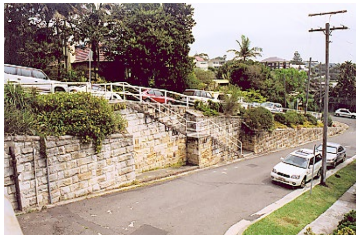
Sandstone retaining wall along Salisbury Street
