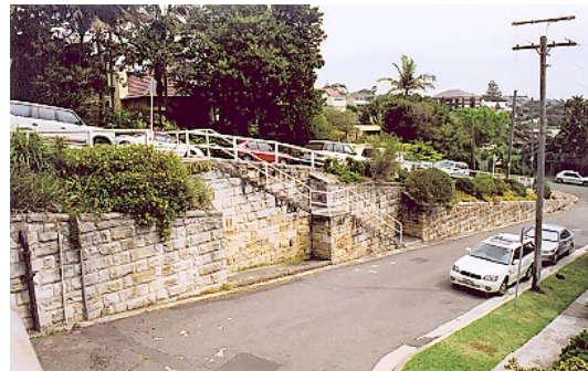
FIGURE 91 Significant sandstone retaining wall
