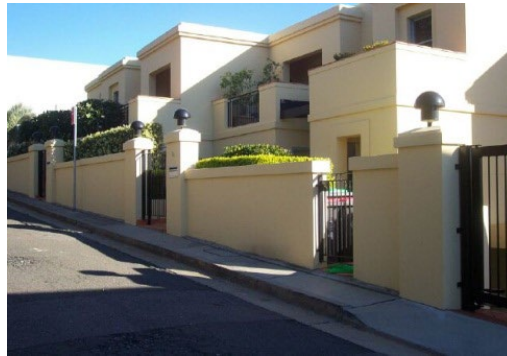
FIGURE 36 Buildings in Gap Road North
