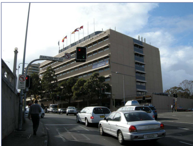
The Edgecliff Centre building
