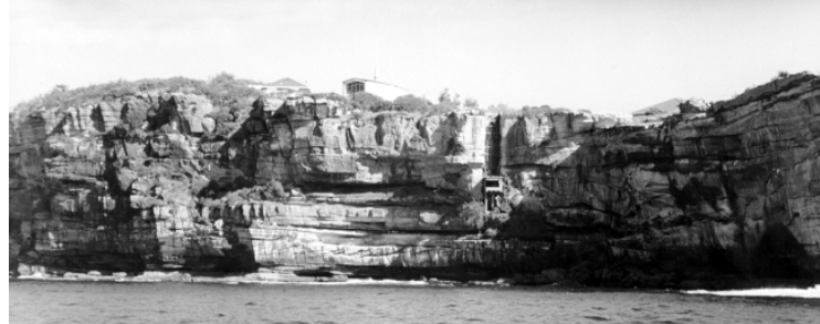
FIGURE 146 The sandstone cliffs that define the precinct on its east side
