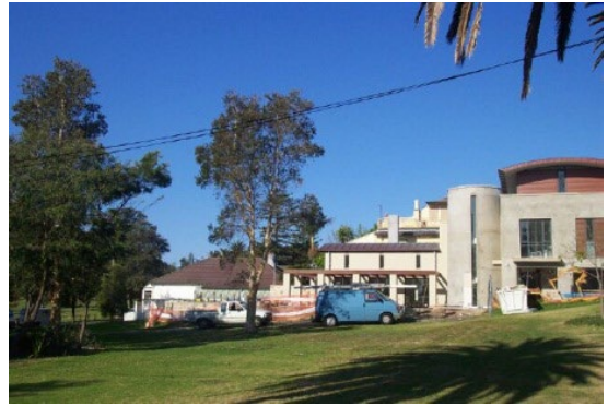
FIGURE 42 View from Robertson Place
