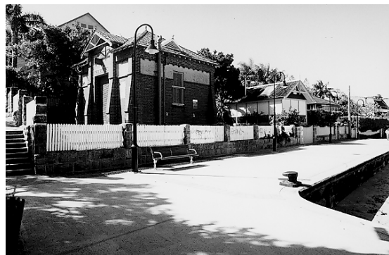
FIGURE 51 Water pumping station at north end of Marine Parade
