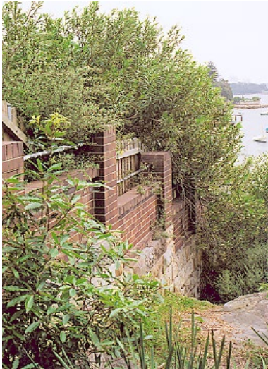
FIGURE 94 Composite wall containing sandstone and face brick on Salisbury Street
