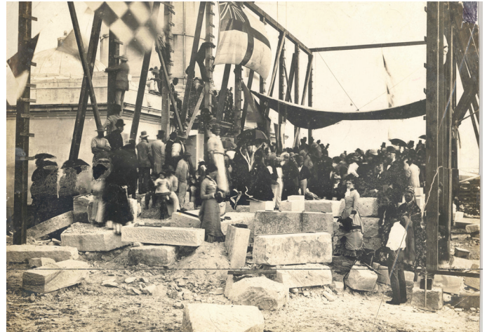
Laying of the foundation stone for the second Macquarie Lighthouse in 1880
