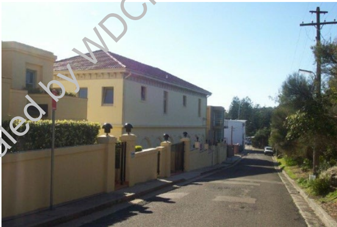
FIGURE 31 Rear of the former Masonic Lodge with residential flats adjacent
