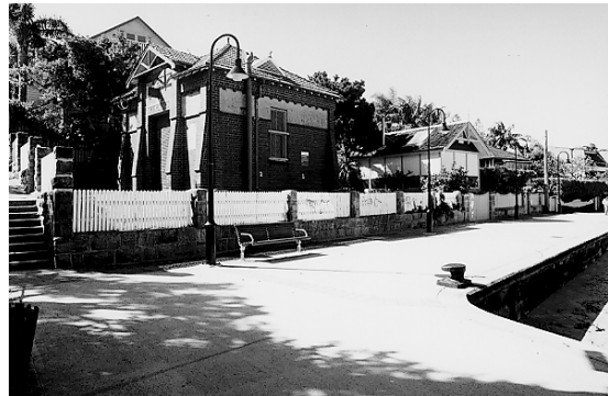
FIGURE 51 Water pumping station at north end of Marine Parade
