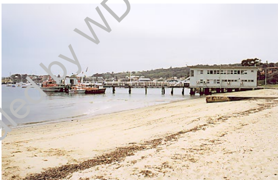
FIGURE 107 Pilot Station at the south end of Marine Parade
