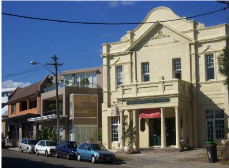
FIGURE 20 East side of Military Road, with former town hall prominent.
