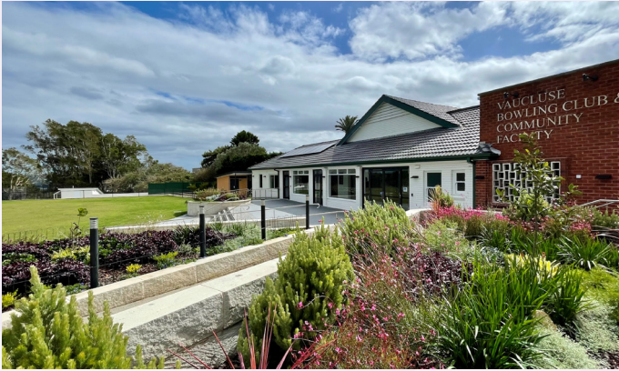
The Vauclose Bowling Club and Community Facility has been renovated and re-opened to the public for hire and new health services.
