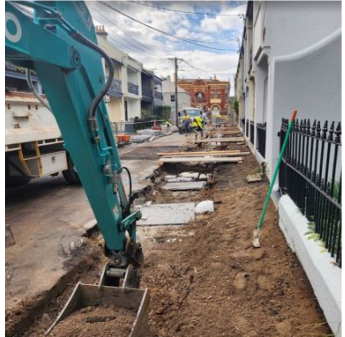
Tunnelling works at George St, Paddington
