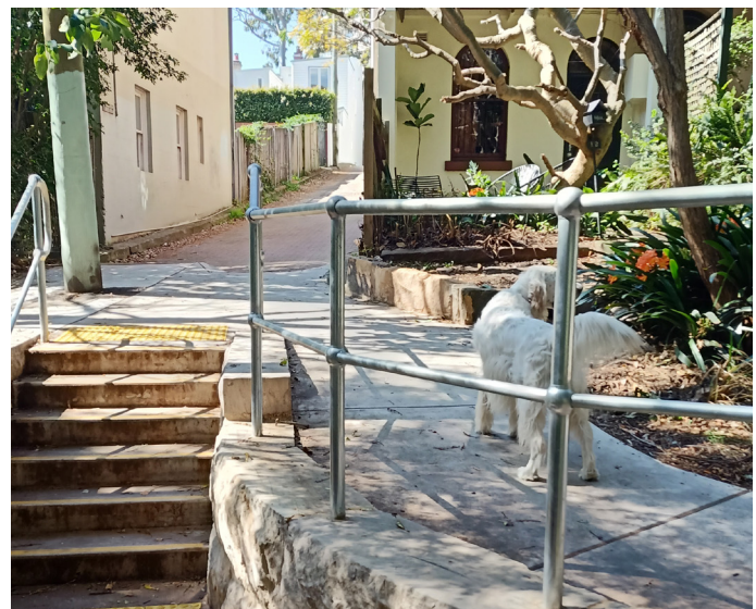
Trumper Park pathway has been upgraded
