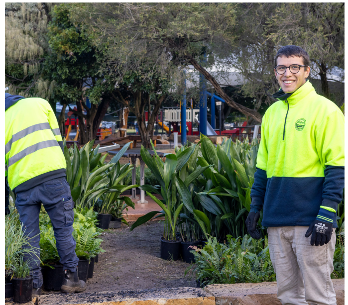
Staff completing planting works at the upgraded Lyne Park playground
