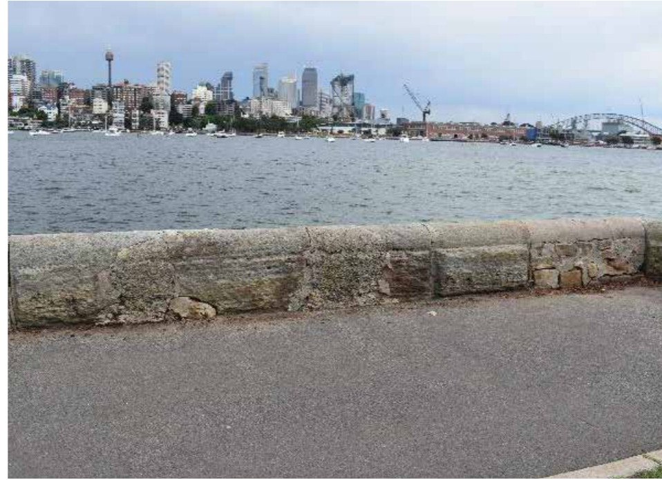
Existing sea wall
