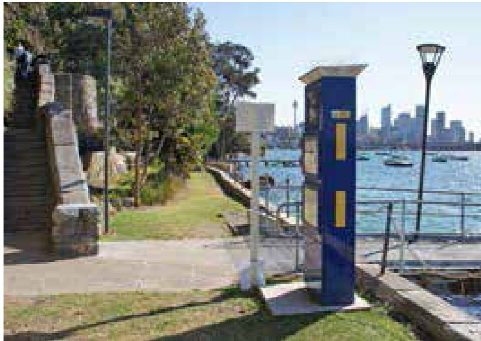
Ferry wharf, turf, foreshore and seawall
