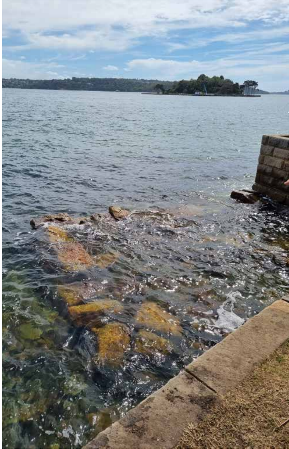
Remains of 19th Century Jetty
