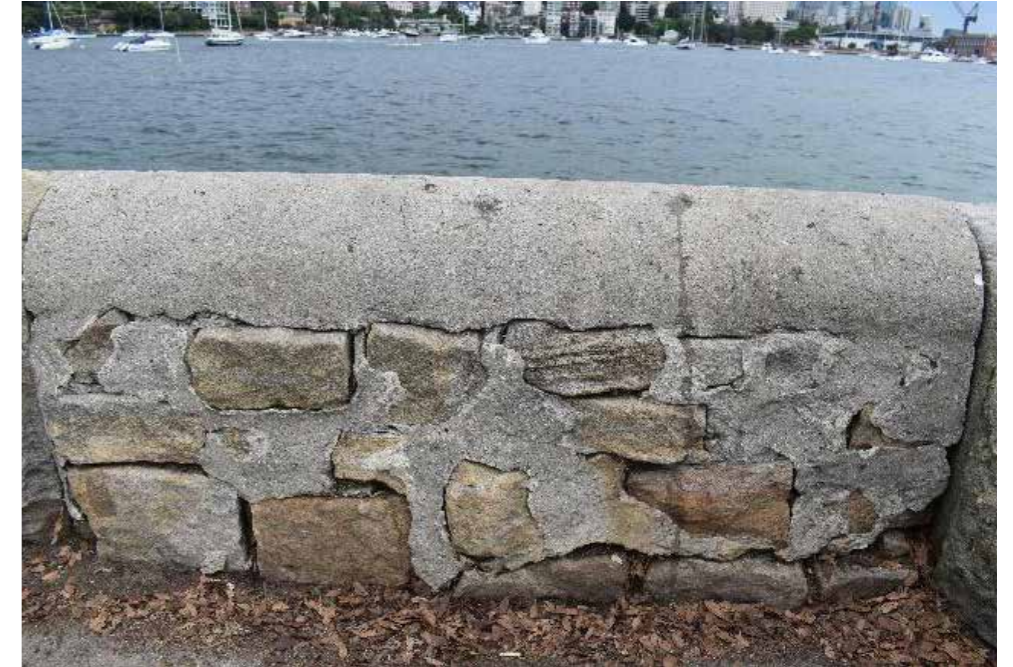
The stone repair to the seawall
