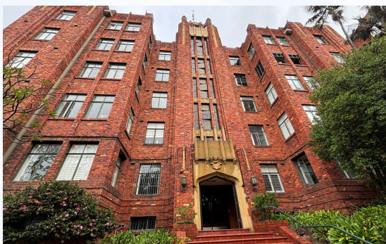
InterWar Flat Building example Hillside, Woollahra
