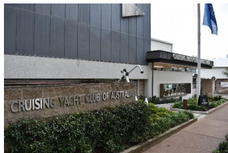
Figure 2.54 The CYCA building beside the footpath of Plantation Reserve. (Source: GML, 2021)
