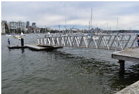
Figure 2.59 The public jetty in Yarranabbe Park. (Source: GML, 2021)
