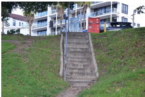
Figure 2.35 Mid twentieth-century concrete stair access in the southeast of the park. (Source: Ari Anderson, 2021)
