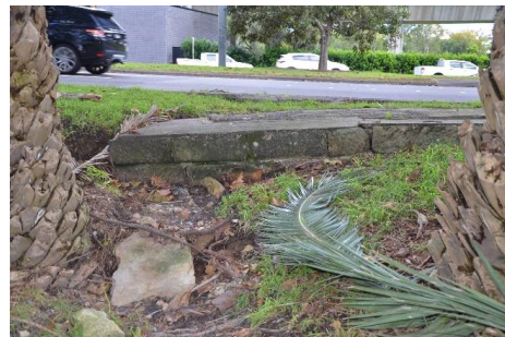
Figure 2.36 Sandstone footing remnants of a tram stop along New South Head Road. (Source: Ari Anderson, 2021)
