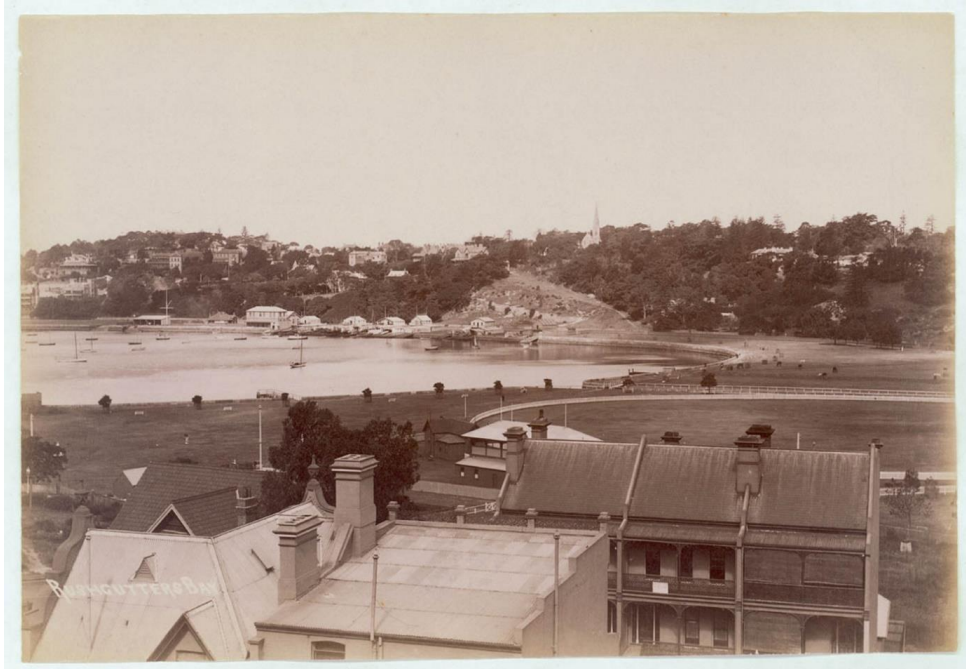
Figure 2.8 View east across Rushcutters Bay showing the oval and some plantings throughout the park, c1900–1910. Boatsheds and development are visible at a distance along the foreshore comprising the present-day Yarranabbe Park. (Source: State Library of New South Wales, a116074h)
