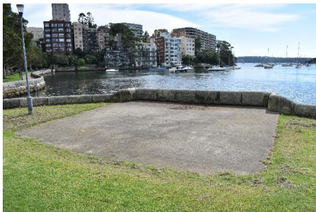
Figure 2.29 An area of hardstand concrete with a modified area of the seawall, below which is a separate outlet.
