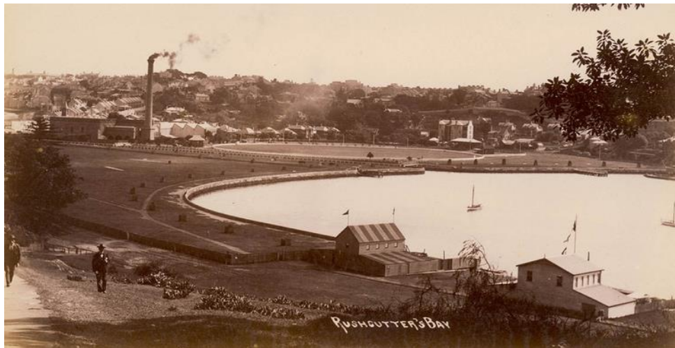
Figure 2.7 View from Darling Point looking southwest across Rushcutters Bay Park, c1900–1910. Tree plantings are visible along the seawall. Boatsheds stand in the foreground prior to the formation of New Beach Road to the north along the western foreshore of Darling Point. (Source: State Library of New South Wales, PXE 711/74)
