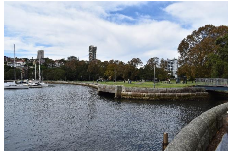
Figure 2.28 The northeast edge of the Woollahra side of Rushcutters Bay Park, showing the stormwater channel outlet in the park.
