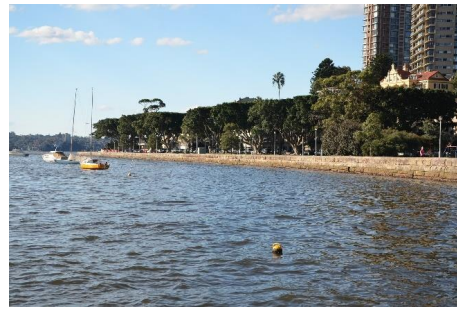
Figure 2.60 The Yarranabbe Park seawall as viewed from the public jetty. (Source: Ari Anderson, 2021)
