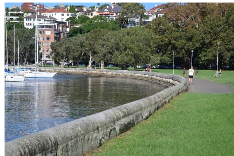
Figure 2.30 The seawall in Rushcutters Bay Park. (Source: Ari Anderson, 2021)
