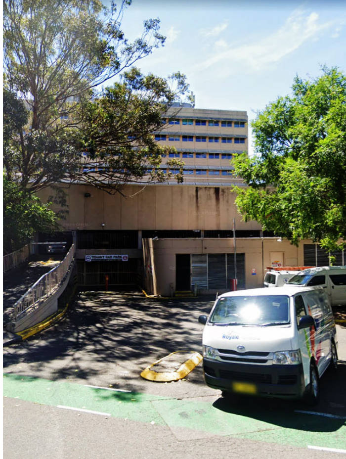
(C) Carpark and loading dock entry point at rear of site
