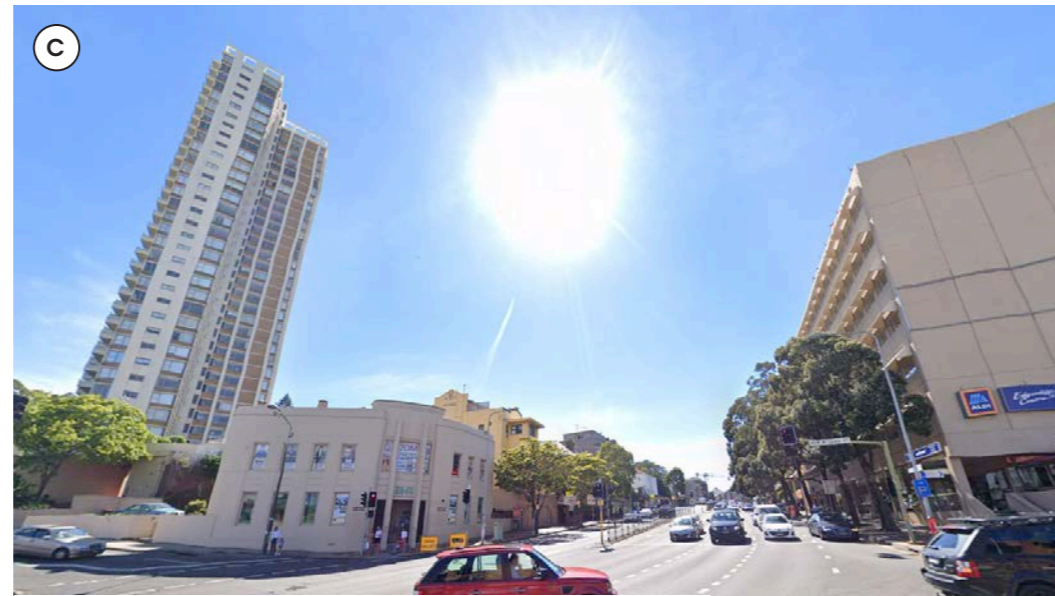
58 New South Head Road - New McLean Street intersection
