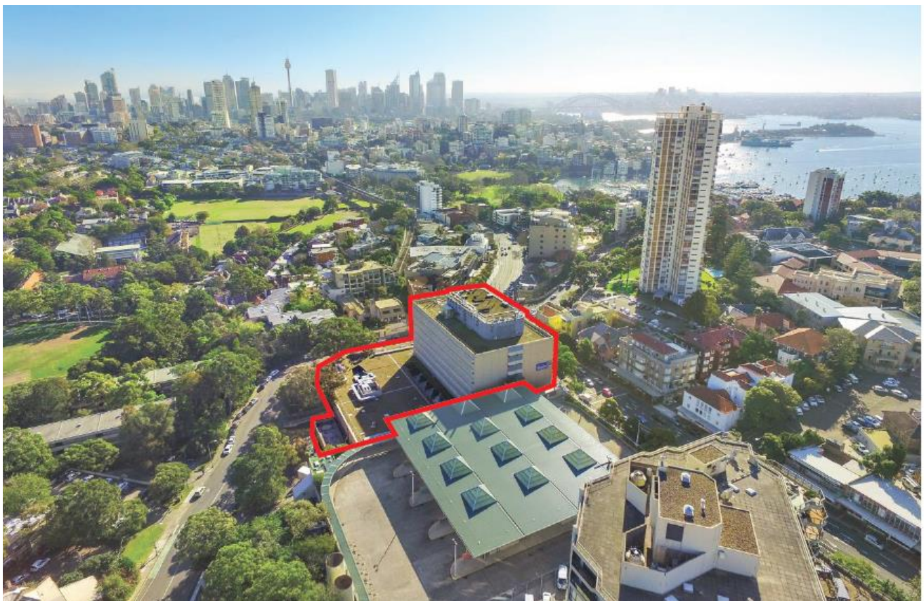
Figure 2 – Site Aerial Source: Nearmaps & Ethos Urban
