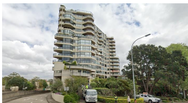
Figure 12 – Eastpoint Tower, looking west from Ocean Street
