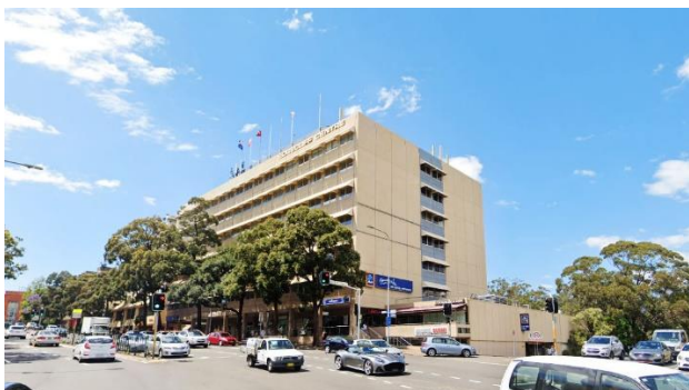
Figure 3 – Edgecliff Centre, viewed from north west
