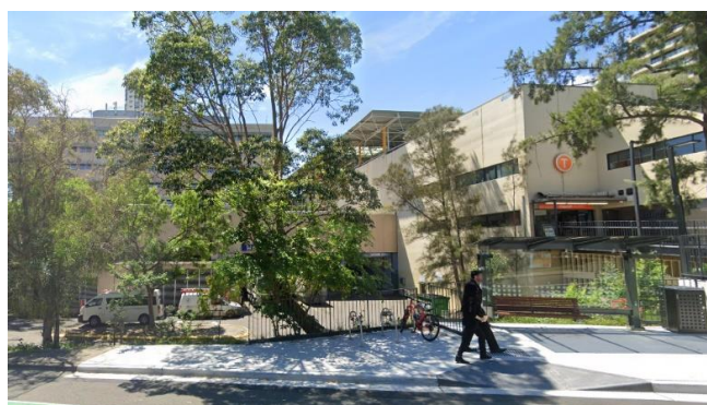
Figure 6 – Rear of the site adjoining the entrance to Edgecliff railway station
