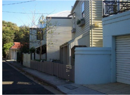
FIGURE 34 Two storey weatherboard cottages on Gap Road
