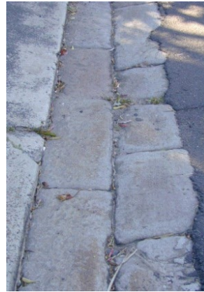
Sandstone guttering
