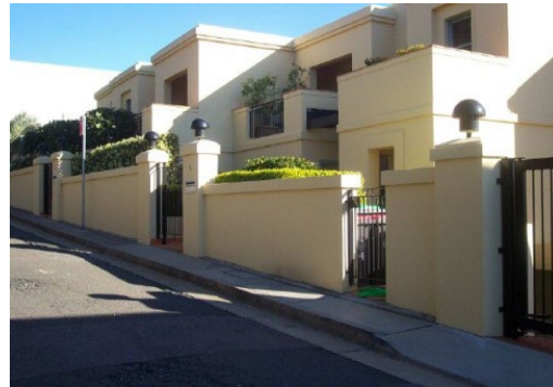
FIGURE 36 Buildings in Gap Road North
