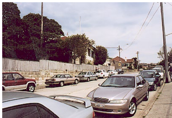
FIGURE 93 Sandstone block retaining wall with traditional timber paling fence above on the east side of Hopetoun Avenue
