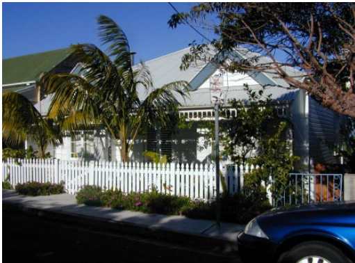
FIGURE 87 Appropriate fencing along Victoria Street
