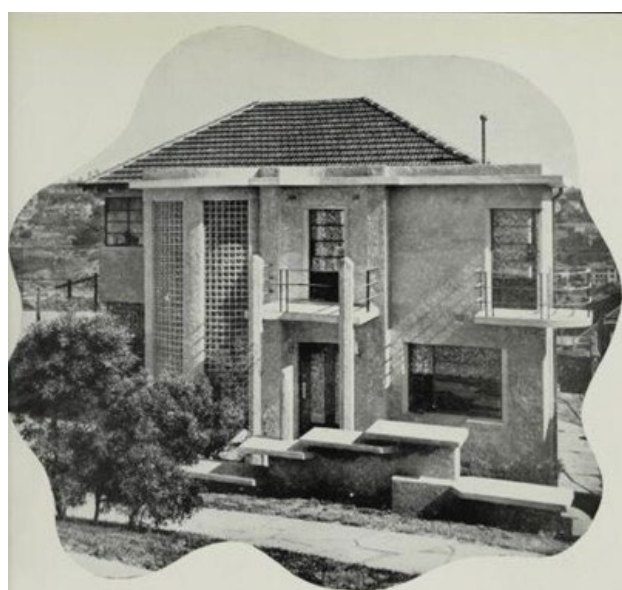
Figure 49 Front exterior of Padova, Streatfield Road, Bellevue Hill, with glass brick stair wall, featured in Decoration and Glass , June 1938 edition under the title 'Australia's First Glass Home'. Architect was Hamlet Agabiti for AO Romano. (Source: Decoration and Glass , 21 June 1938, p11)
