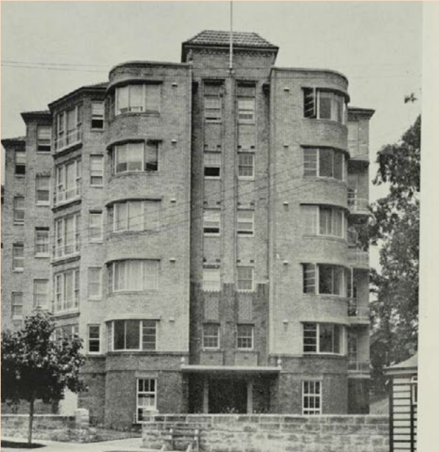
Figure 41 Edgecliff House, 127 Ocean Street, Edgecliff, 1937. Demolished in 1971 to make way for the eastern suburbs railway. (Source: Building , Vol 61 No 364, 24 December 1937, p 45)
