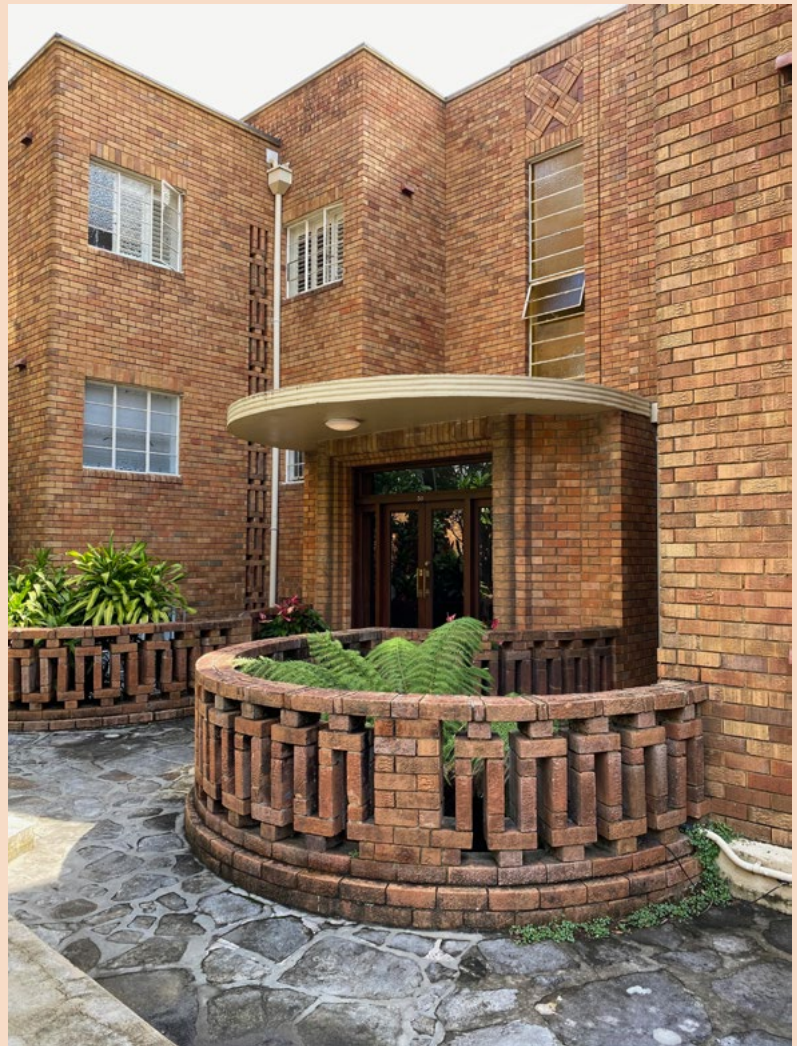
Figure 46 The entry to the lower buildings, showing the restrained palette with much of the detailing achieved through brickwork.
