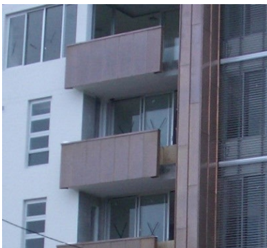
FIGURE 3 Part projecting balcony
